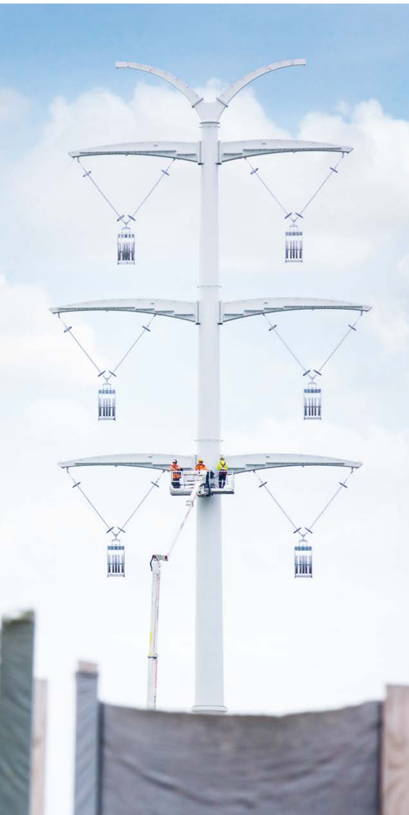
Novel design: between Millingen substation and the Dutch border Amprion is trialling a new type of pylon.
