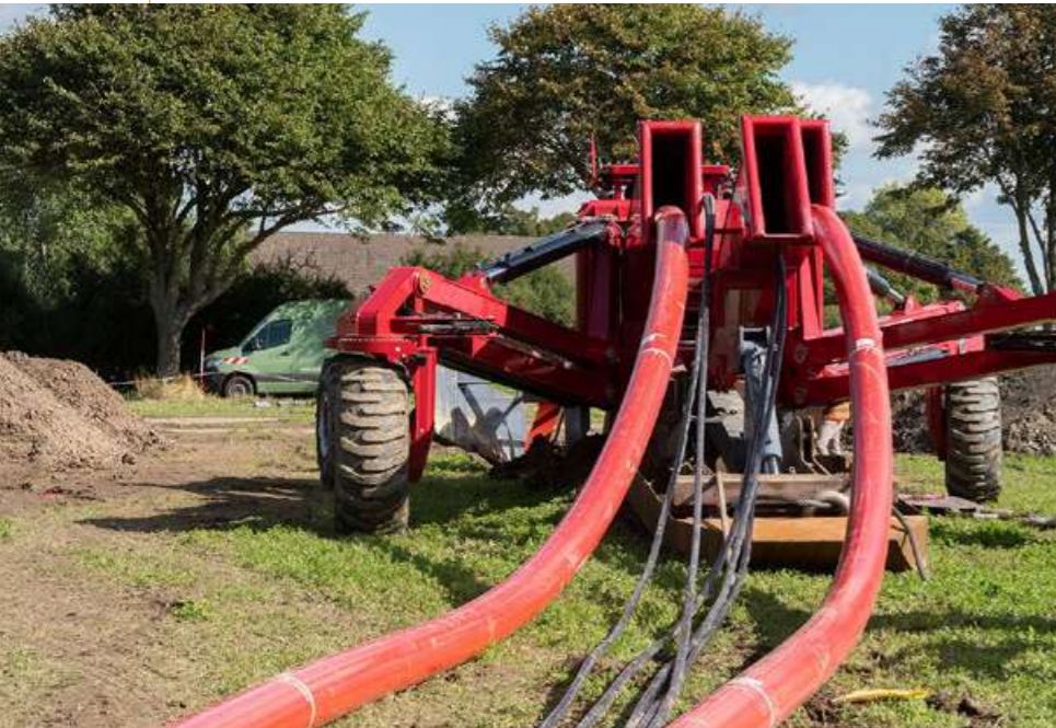
FIG. 25 Two-blade cable-laying plough during the Amprion test
