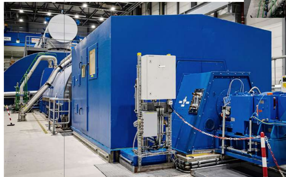
FIG. 14 AND 15 Rotating phase shifters with a start-up converter at the Westfalen E power plant
