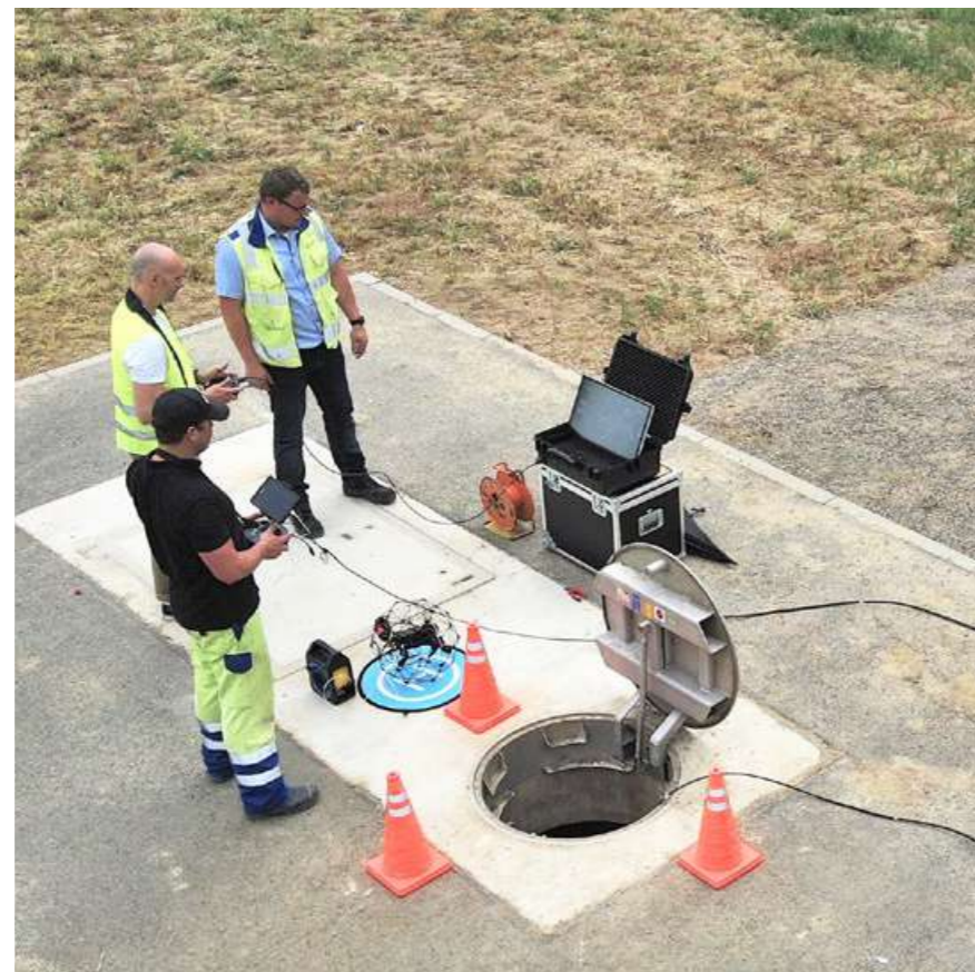
FIG. 41 Inspection of a 15-metre-deep cable pit with an indoor cage drone
