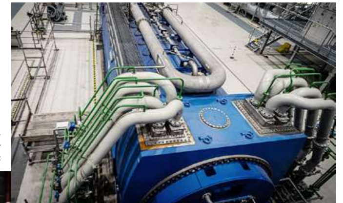
FIG. 14 AND 15 Rotating phase shifters with a start-up converter at the Westfalen E power plant
