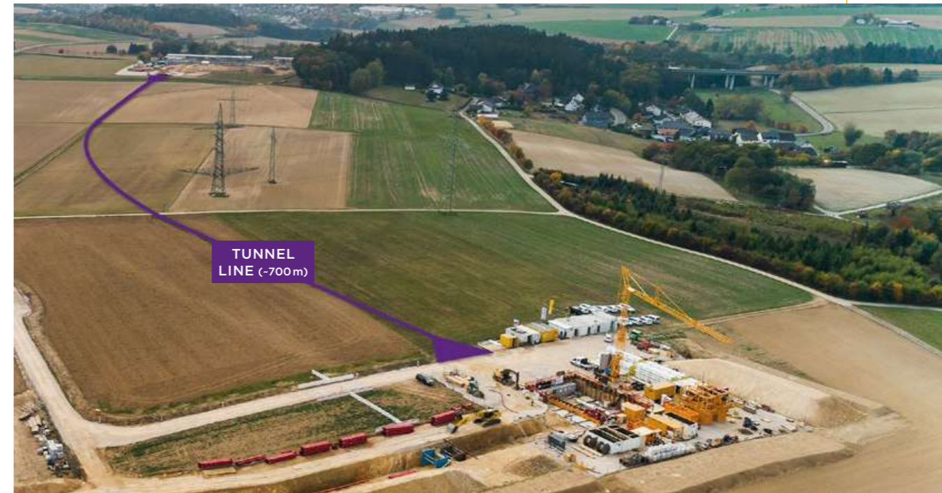
FIG. 24 Amprion GmbH E-Power-Pipe construction site in Bacharach
