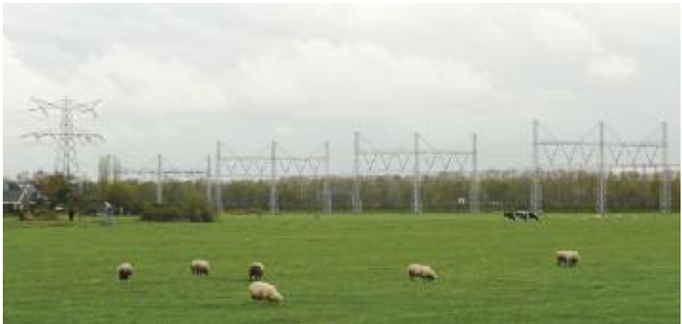
Figure 2: A 380-kV line with lowered conductor wires hanging from portals in a single horizontal plane to minimise the collision risk for Great Cormorant, Eurasian Spoonbill and Purple Heron that traverse this stretch of line every day while commuting between their breeding colony and foraging areas (Muiden, the Netherlands).
